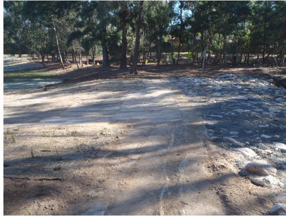
A RECENT ADDITION & JUST COMPLETED IS A STONE & ROCK SPILLWAY LEADING INTO THE RETENTION BASIN. THE SIDES HAVE BEEN PEGGED USING HESSIAN THEN PLANTED OUT. THE WATER FLOW IS FROM THE RIGHT AND FLOWS INTO THE BASIN TO THE LEFT. THE ROCKS REDUCE WATER VELOCITY.
